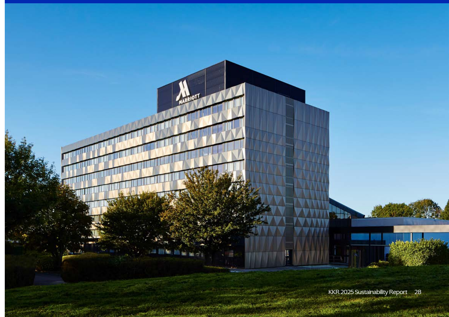
Hospitality asset in Portsmouth, United Kingdom.
